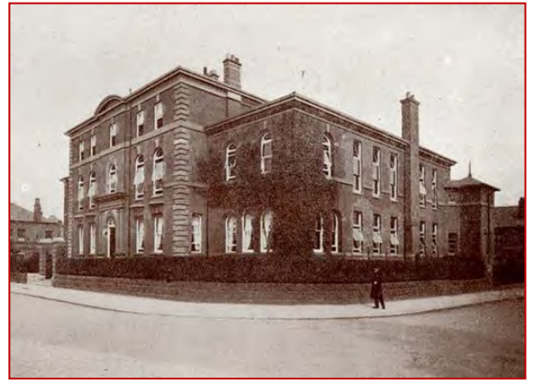
Altrincham General Hospital as it appeared in 1914, following the extension on Regent Rd to the original 1870 building, designed by local architect Peter Pons.
